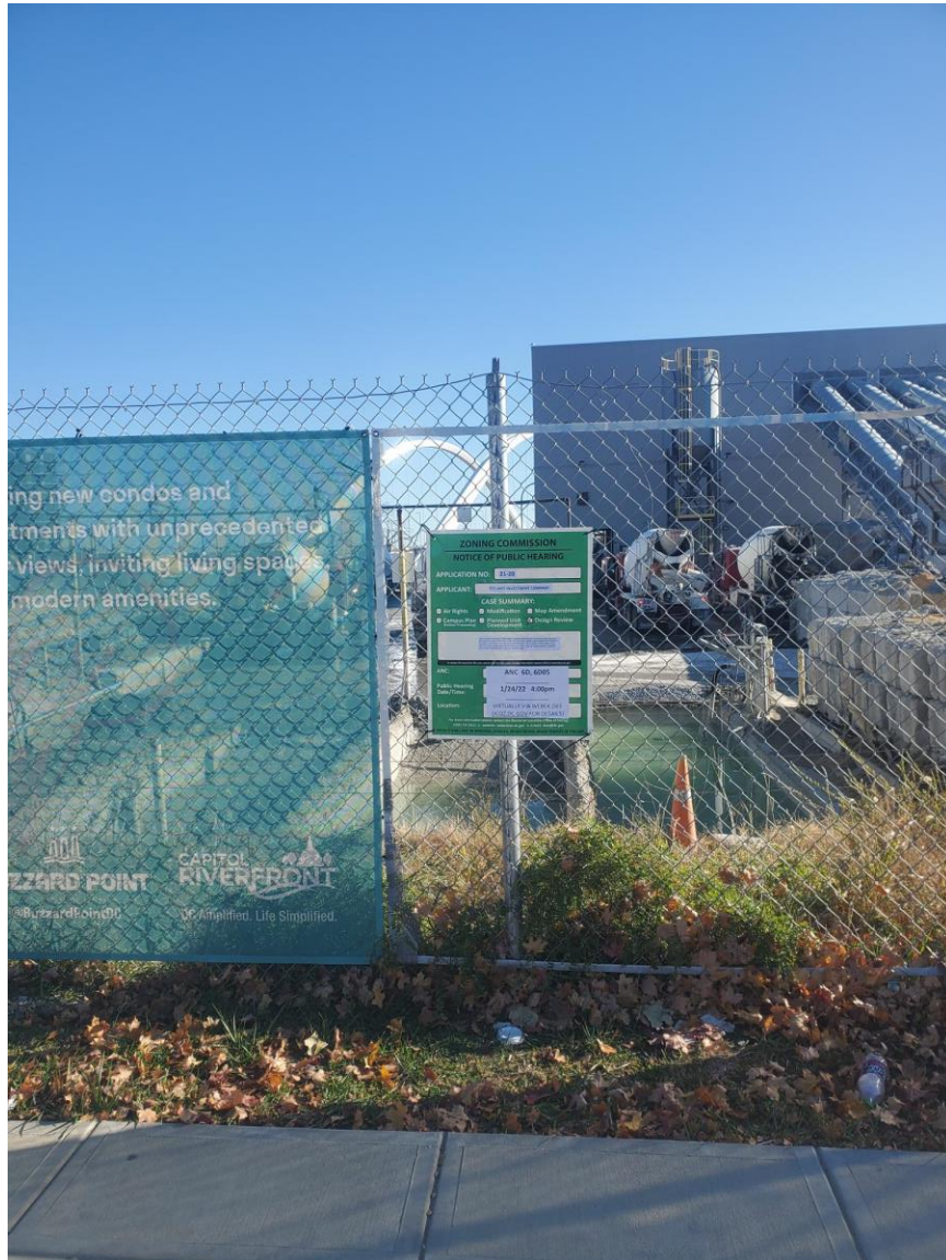
Figure 1 - Placard / Sign #1 – Half Street, SW – Installed 12/13/2021
